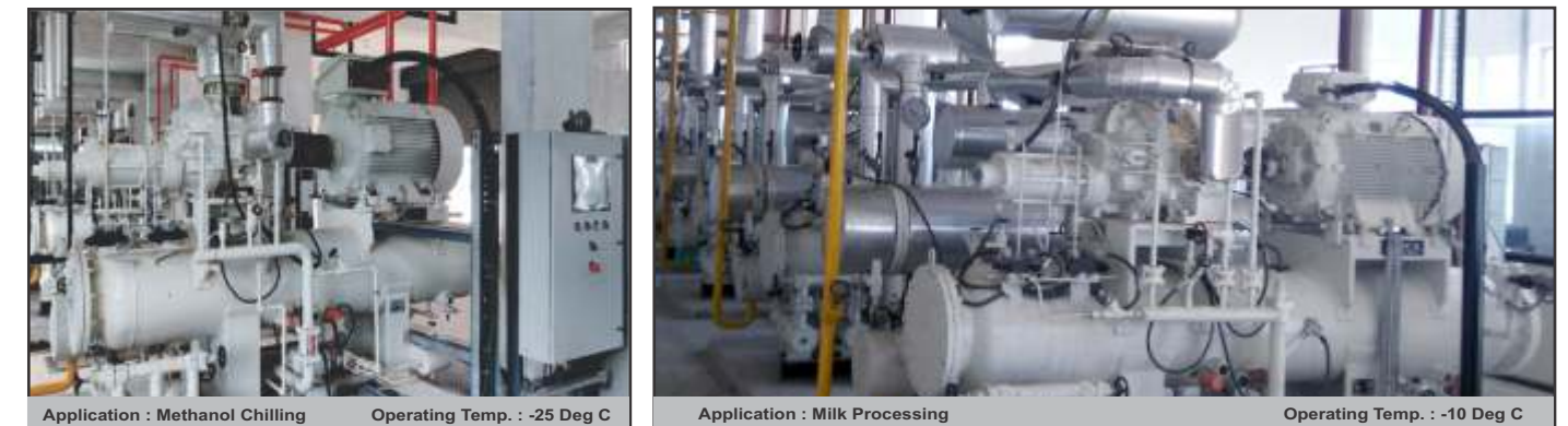
Application : Methanol Chilling Operating Temp. : -25 Deg C
